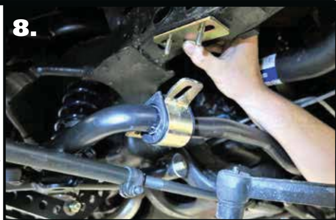
8. Install the bushing strap over the swaybar bushing with the wide side of the strap to the inside on the car. We found some steering box conversions hang down further than others. If yours happens to hit the sway bar, add a 2nd spacer under the bushing. a 2nd set of spacers along with longer hardware is supplied in this kit.
