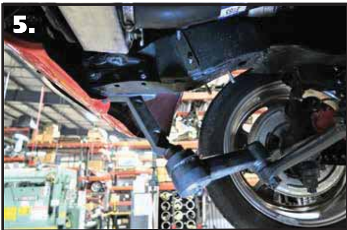
5. Disconnect the idler arms from the frame.
