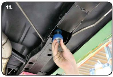
**11.** Push the front subframe connectors up against the OEM subframe. Reinstall the OEM body bushing/bolt.
