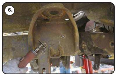
6. The OEM upper coil spring and I-beam mounts need be removed from the frame rail. This can be done by either drilling the rivets out or removing the rivet heads and driving them out. We remove the rivet heads by cutting a " + " in the head with a die grinder then we cut the head off with a hammer and chisel or with an air chisel. Once the head is removed, the rivet can be driven out with a hammer and punch.
