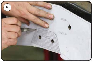
**6.** Use the template to center punch the corner holes of the area that needs to be cut out.
