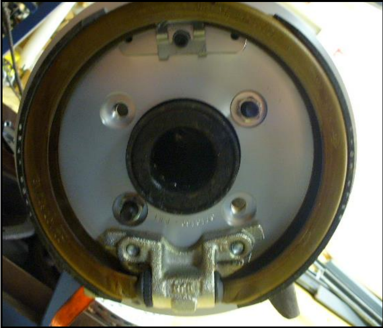
Park brake assembly correctly installed
